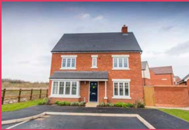
Great Denham, Bedfordshire
